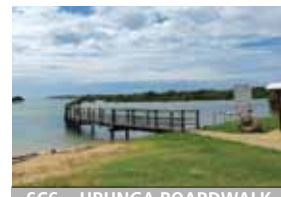
SC6 – URUNGA BOARDWALK
